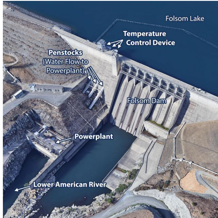
Location of the existing temperature control device and other nearby features at Folsom Dam (USACE)
