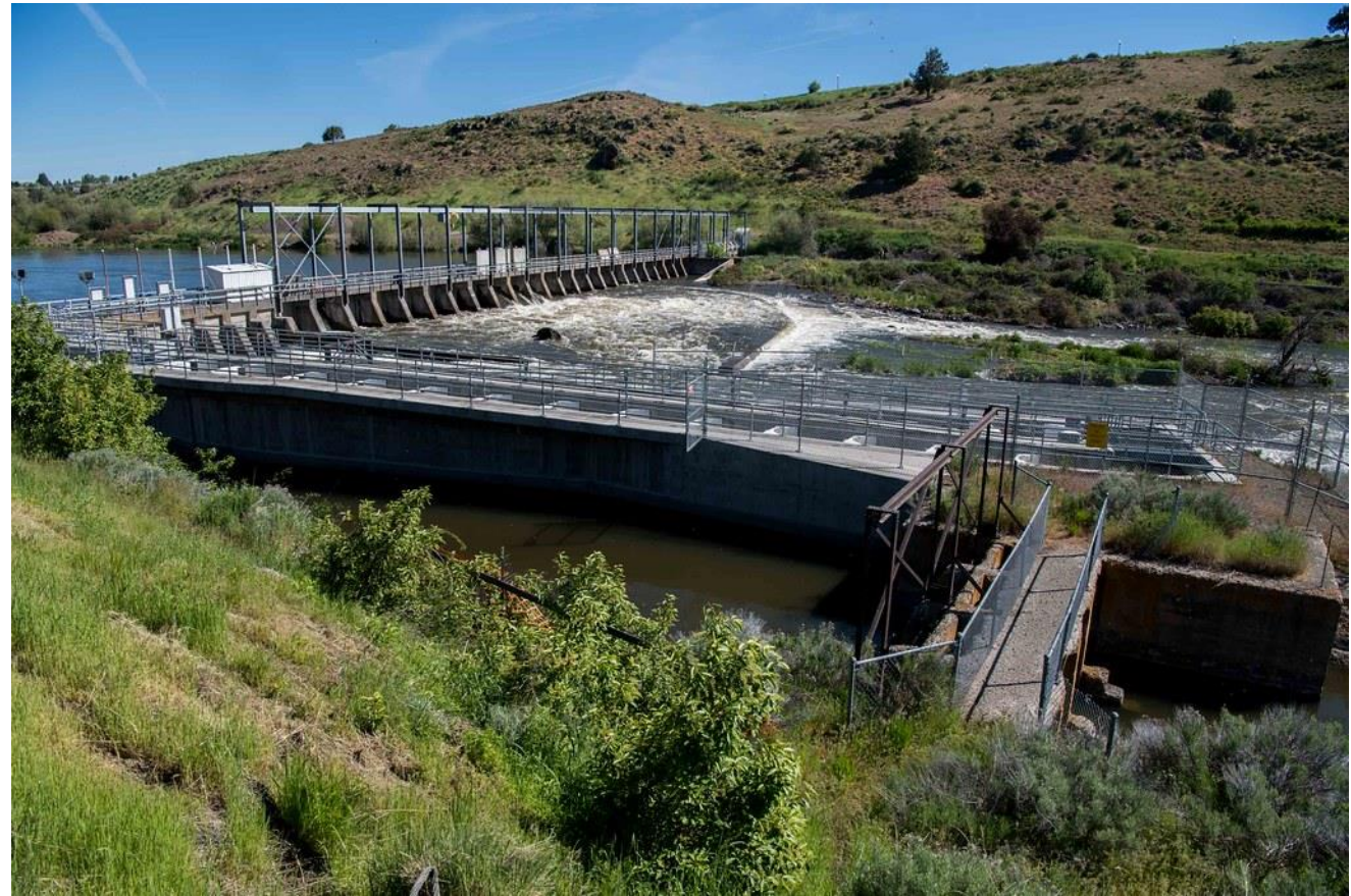
Bureau of Reclamation
