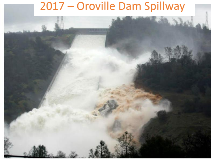
Water flows through a break in the wall of the Oroville Dam spillway Feb. 9, 2017, in Oroville, Calif. AP PHOTO/RICH PEDRONCELLI
